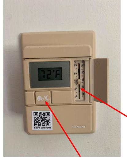
Occupancy button, push this button to put the room into an occupied mode for 12 hours. Pushing the button at any time will reset the counter to 12 hours.
