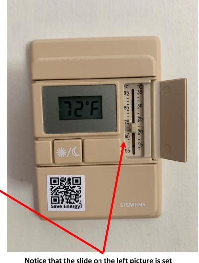
Notice that the slide on the left picture is set for 75. Because 72 is the warmest setting, this thermostat will control to 72 degrees. The slide on the right picture is set for 71. This thermostat will control to 71 degrees.
